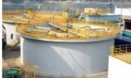
Clarifier of Water Treatment Plant
