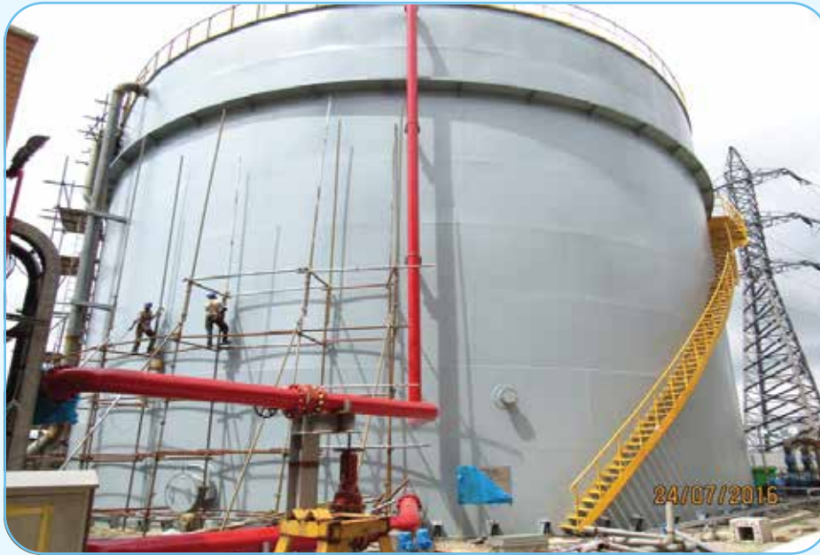
Clarified water storage tank (paint working)
