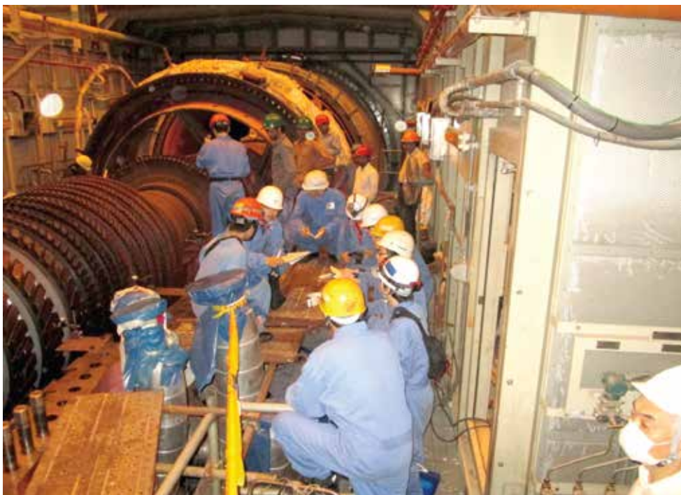
Gas Turbine Rotor Run out Checking
