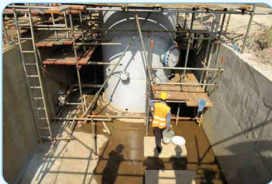
HRSB (grouting work)
