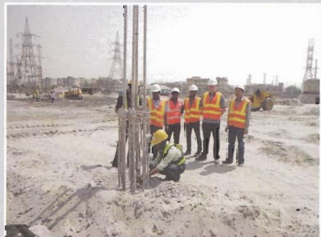
Soil Integrity Test of Siddhirganj 335 MW CCPPP
