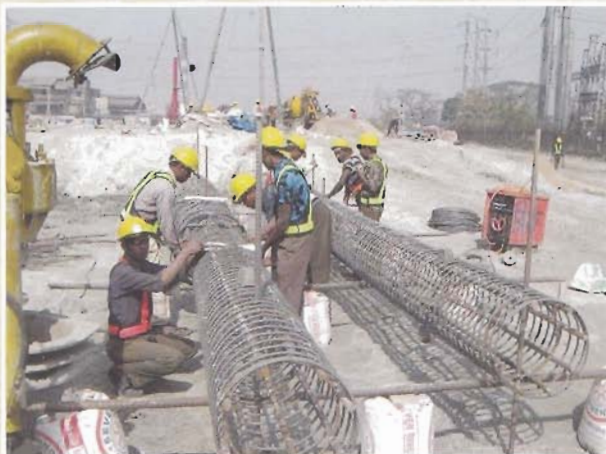
Siddhirganj 335 MW CCPPP
