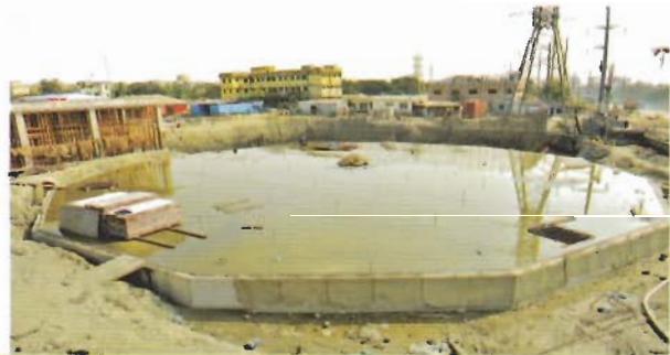
Civil work for Siddhirganj 335 MW CCPPP
