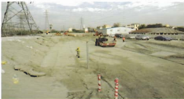
Land preparation for Siddhirganj 335 MW CCPPP
