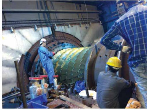
Turbine inspection plus of Gas Turbine
