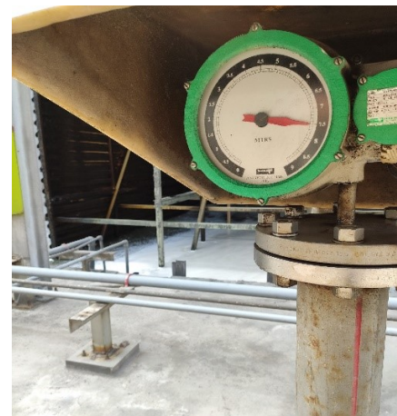
Fig: Photos of installed gear type level transmitter in cooling tower basin.
